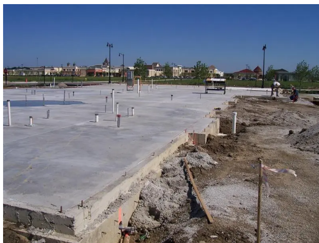
Mistakes will be cast in concrete, literally. Forgotten items are expensive to recapture. (Courtesy of Wayne Usiak)
