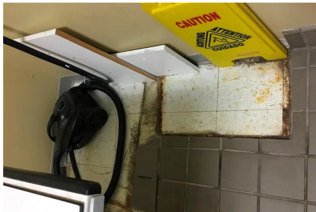
Trying to hide a urine problem in vinyl tile by installing porcelain tile over it. (Courtesy of MD Architects)
